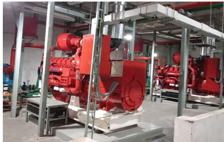
Diesel Generators
